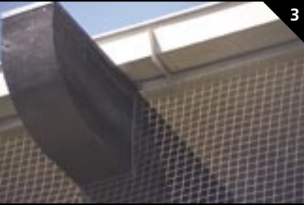
1) A strong perimeter cable holds the black 3/4" StealthNet tightly against the wall in a parking structure. 2) StealthNet supported on telescoping poles (p. 28) completely excludes birds from all the rooftop equipment. 3) StealthNet protects an opening on the front of an office building. Notice the attention to detail which insures a completely bird-free system.
